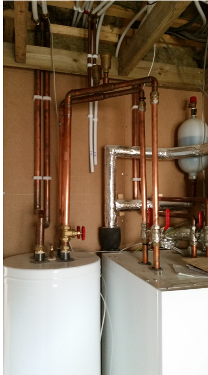
Worcester Bosch heat pump and buffer tank
