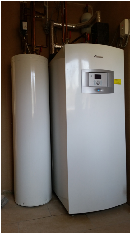
Worcester Bosch heat pump and buffer tank
