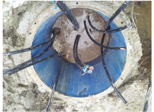
Boreholes waiting manifold connection
