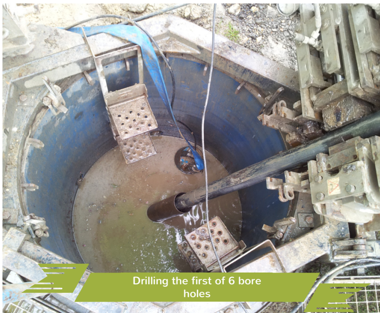
Boreholes being drilled
